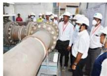
The new Oxygen PRMS (Pressure Reducing and Metering Station) of capacity 84000Nm3/hr has been installed to fulfill the oxygen demand for modernization projects like Converter- C & Caster-3 of SMS-2. Besides, the new system will ensure 100% avail-
